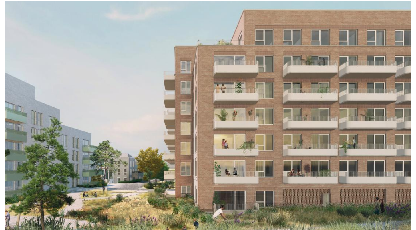
Fig.33 View down county boundary towards the west, with views of the balconies on Block A2
