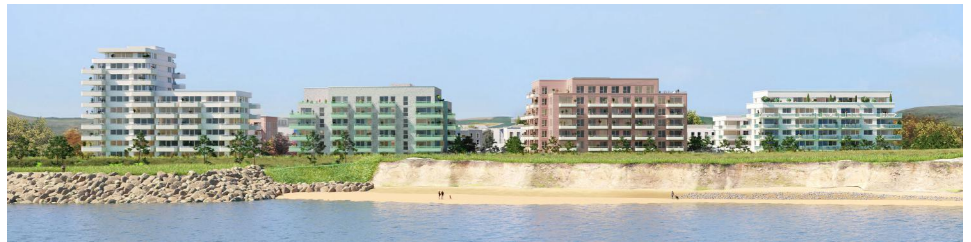
Fig.8 View of Block A & B looking west from the bay
